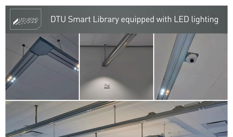
Today DTU Smart Library acts as a living laboratory where students and scientists spend time and test new technologies. The lighting is no exception. Here, the numerous traditional light fixtures have been replaced with custom made LED luminaires, which vary the colour temperature as well as light intensity depending on user needs and time of the day.
