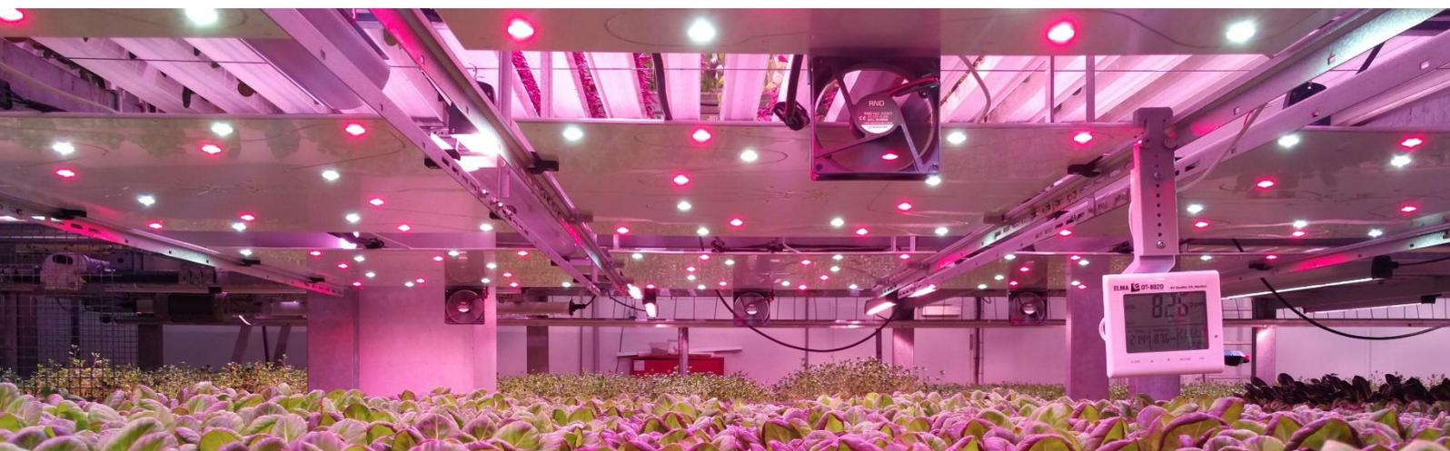
Choosing the right spectrum for specific plant is essential for crop yield but it is also a question of ensuring that the electrical energy used to drive the growth light panel is used optimally by generating light photons with the highest impact on plant growth and thereby crops produced with the right quality. The optimal spectrum will increase the yield.
