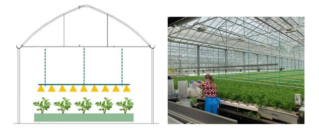
The rails are light weight (aluminum) and allow for flexible configurations in terms of size (growth areas to cover) and spacing between the TRACY® Horticulture growth light panels. The TRACY® panels are mounted fast and easily with click-on brackets attached on the rails.
