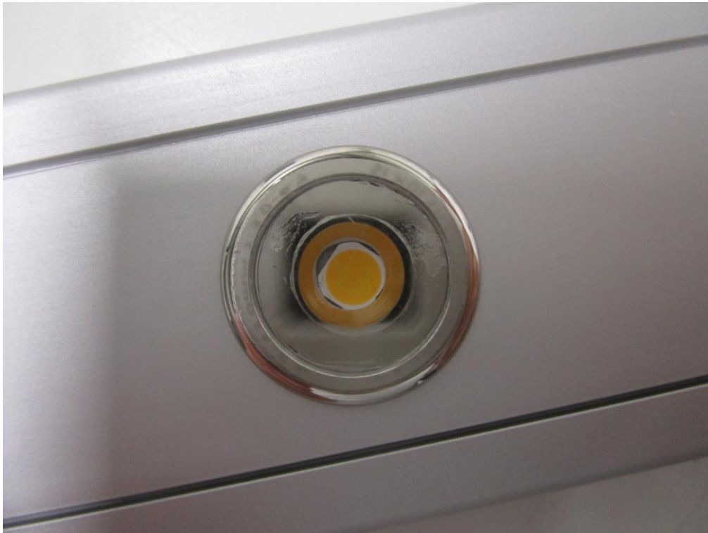
Photo 5 Visual inspection. IP6X. No dust observed inside LED sockets.
