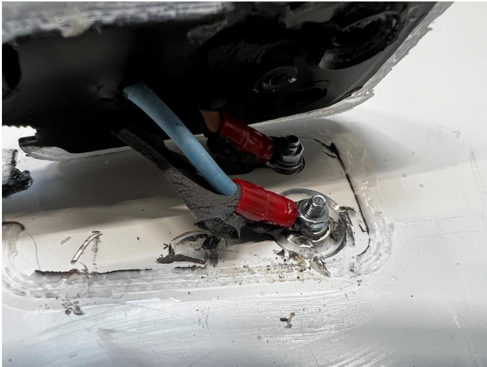
Photo 36 Visual inspection, IPX7. No Ingres of water observed inside power connection.
