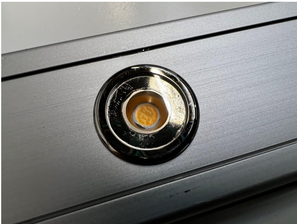
Photo 27 Visual inspection, IPX7. No ingress of water observed inside LED socket. Similar for all LED sockets.
