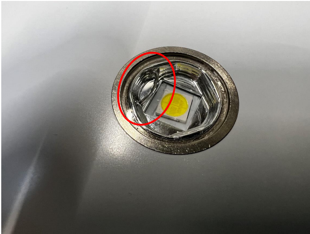
Photo 32 Visual inspection, IPX7. Ingres of water observed inside LED socket (numbered 1 on overview photo).
