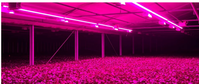
Figure 4 Light distribution from 4 HORTISABER lamps (6m long) – grow bed covered is 12m long and 6.7m wide.
